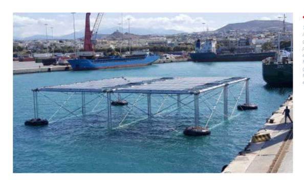
The floats move up and down in rhythm with the waves, generating electricity. Smaller plants are recommended as emission-free replacements for conventional diesel generators, for an aquaculture facility with a self-sufficient energy supply for example.
